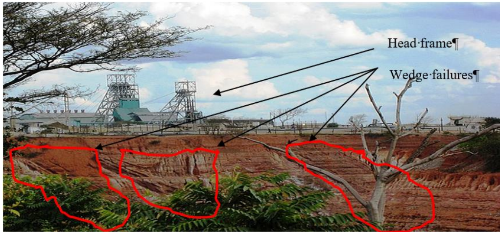
Fig. 2: Nkana open pit Area K wedge failure
