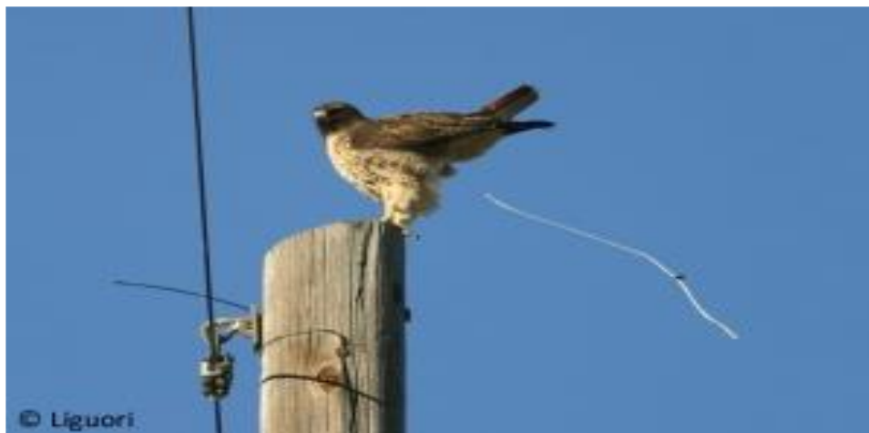
Figure 3: Birds as one of the causes of dips on the transmission network (Source: Rens, 2022).
