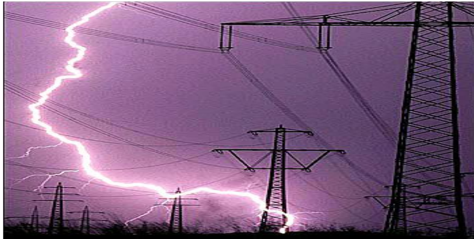
Figure 2: Lightning as one of the causes of dips on the transmission network (Source: Rens, 2022).
