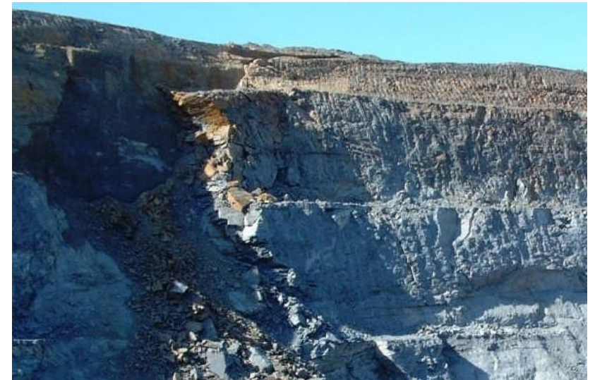
Wedge failure at Round Hill Open Pit- New Zealand (Brown I 1996)
