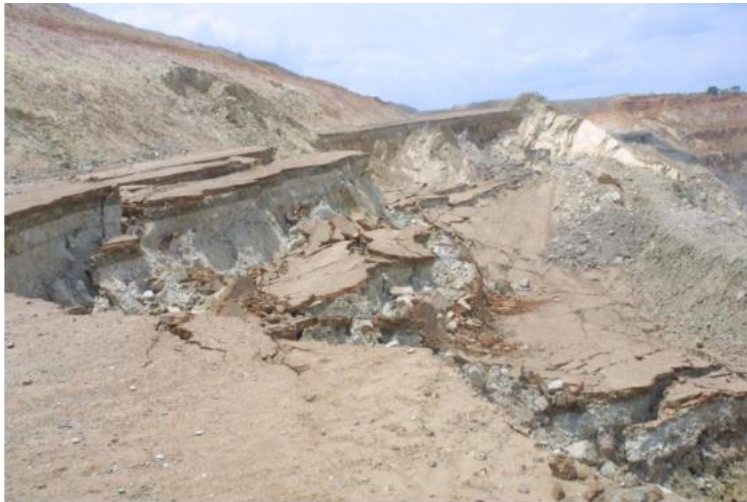
Wedge failure at COF&D- Zambia- Bowa and Kasanda 2020
