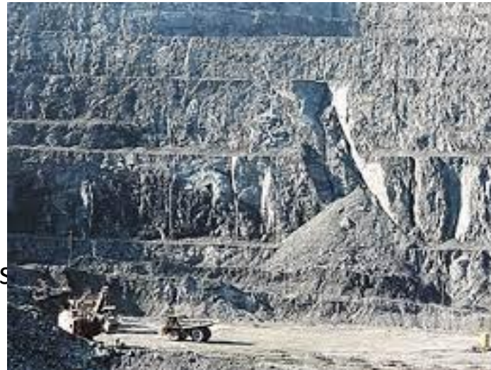
Wedge failure at Kargoorlie mine- Australia- Makarov et al. 2022
