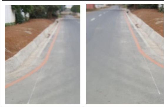
Figure 3: Orange edgeline used instead of accepted yellow edgeline
