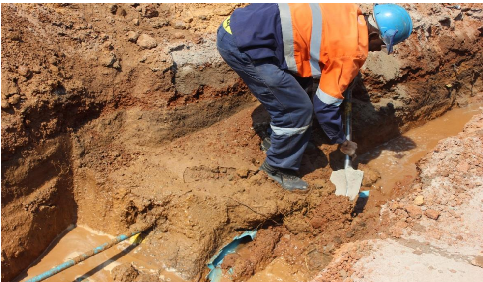
Figure 1: Broken pipe due to lack of excavation clearance from the utility (Mufalo, 2016).
