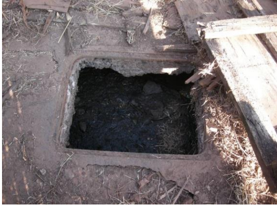
Fig 3: Dry and abandoned septic tank
