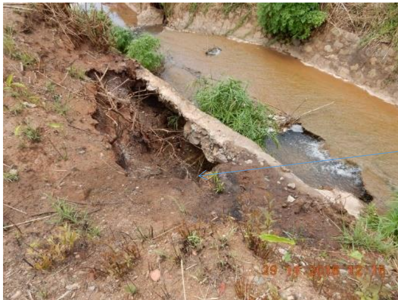
Figure 3.5: Water Discharge in Cracked canal
