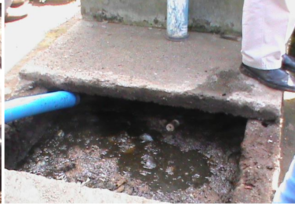
Fig 4: poorly maintained septic tank
