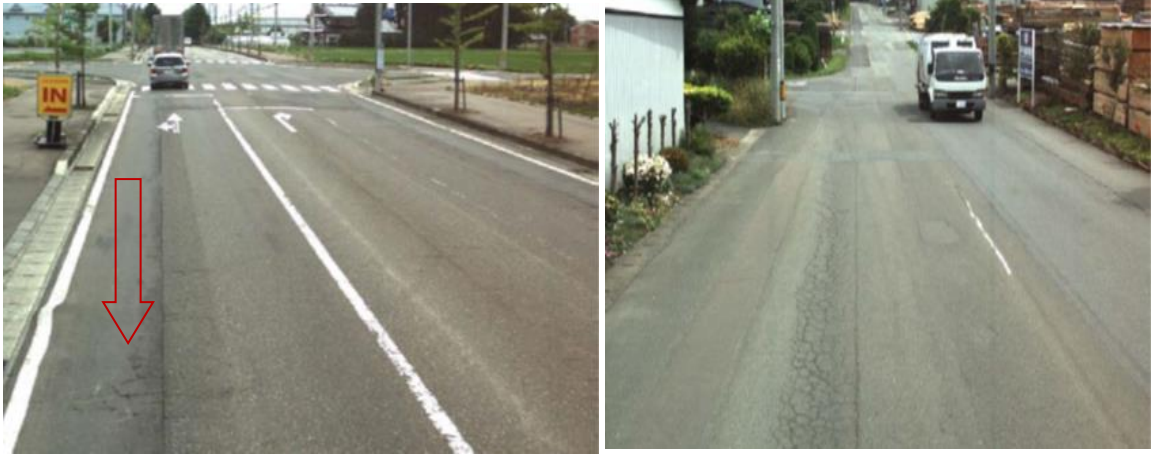
Figure 4: Correlation between road surface conditions and IRI (IRI=11 ~ 12): A condition that the paved road has already been eroded and it has resulted in a series of potholes.
